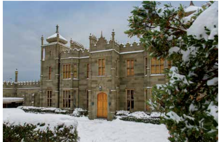
Vorontsov Palace. The south facade Photo courtesy of the Alupka Palace and Park Museum-Reserve
