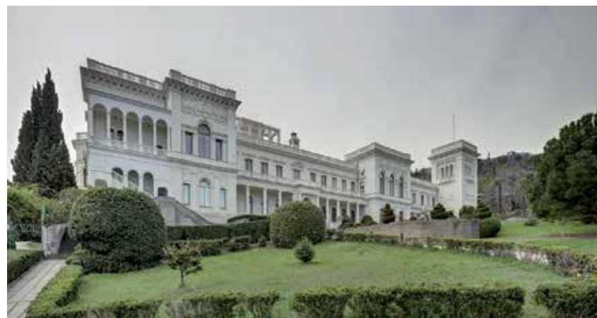
Livadia Palace. The east facade Photo K. Postnikov
