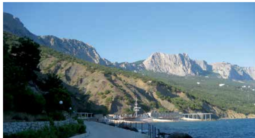
The eastern boundary of the territory of the Mellas sanatorium. In the foreground is a gravitation embankment bordering a landslide tongue with a park and sanatorium buildings located on it. The foundation of the embankment is formed by a landfill of imported limestone rocks; an esplanade was arranged above the landfill which protects the landslide deposits from being washed away and loads the frontal part of the landslide. Photo V.I. Myslivets
