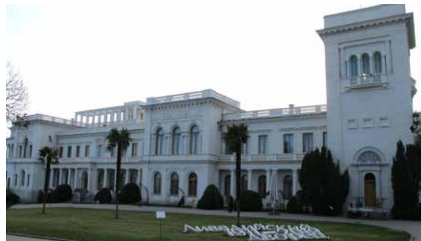
Livadia Palace. The east facade Photo K. Postnikov
