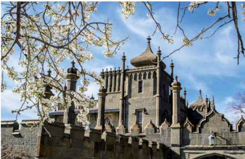
Vorontsov Palace. Roofscape Photo courtesy of the Alupka Palace and Park Museum-Reserve
